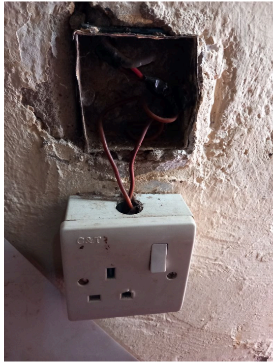
FIGURE 2: Examples of unsafe practices captured during wiring inspections.
